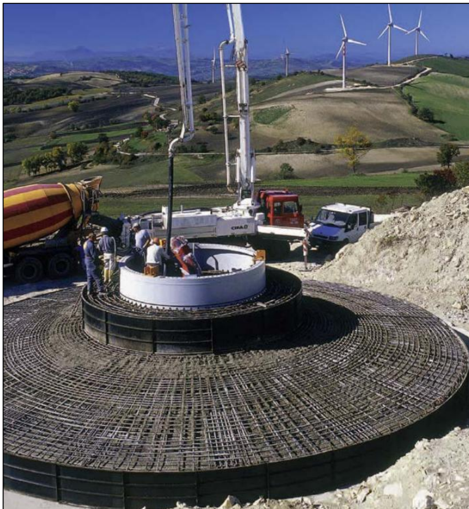
Plate 3.3: Wind Turbine Foundation 4
