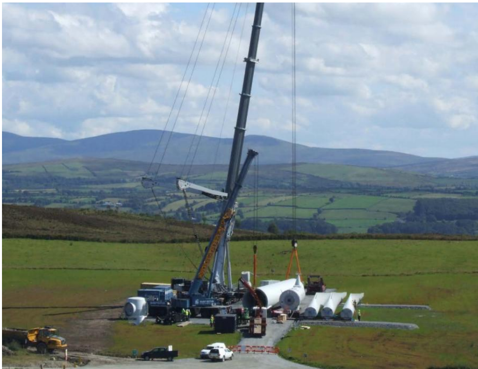
Plate 3.4: Wind Turbine Erection 7
