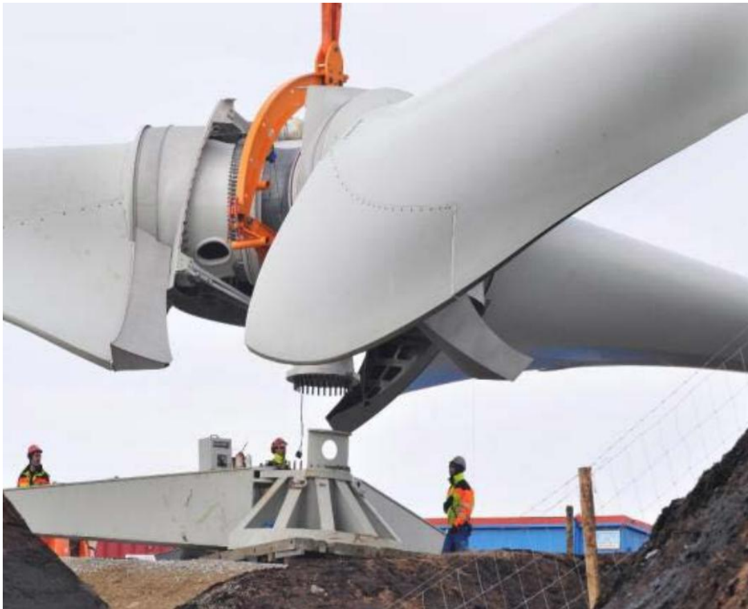
Plate 3.5: Assembly of Wind Turbine Blades 7
