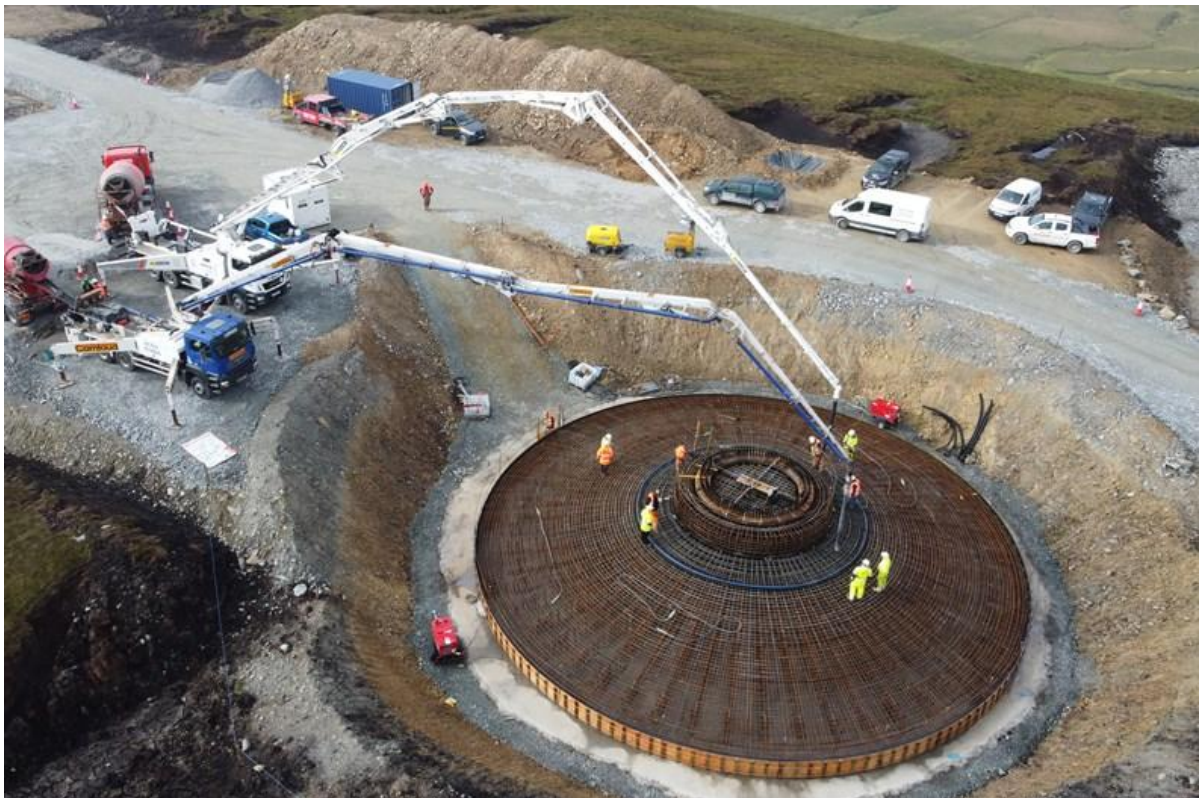
Plate 3.2: Turbine Foundation under Construction with Adjoining Crane Pad 3
